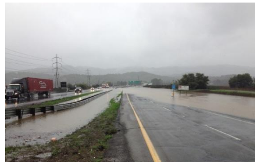
Exhibit 4: Novato Creek Flooding During Closure Prior To 2017 Repairs
